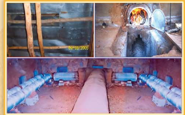
Energy saving intervention - Integrated barn designed (2001)
