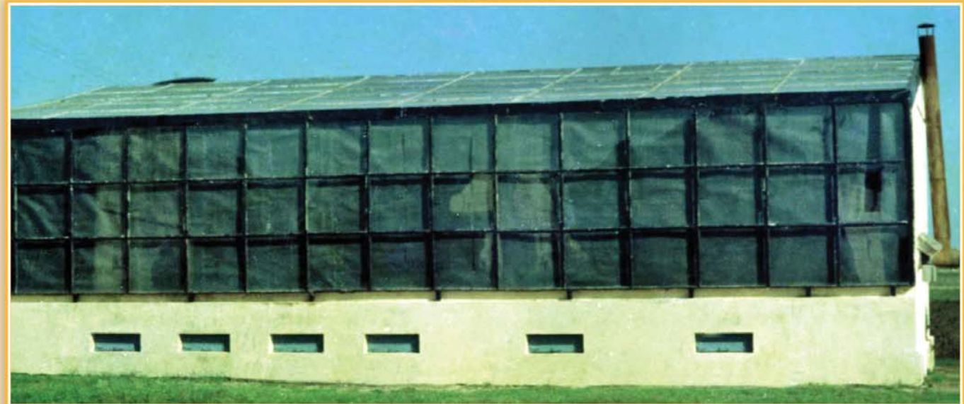
Use of solar energy for curing initiated (1985)
