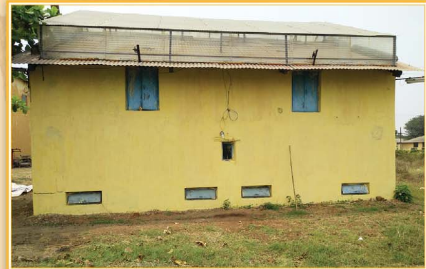
Solar energy intervention - Polycarbonate roof chamber recommended (2021)
